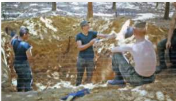
Troops digging Operations bunker in rubber trees.
